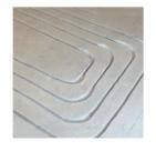
Our specialist machines effortlessly mill or cut a neat 18mm groove in virtually any screeded floor. The pipes are located just below the top of screed and hence provide an exceptional response time with perfect level of comfort and warmth. Radiators can be removed and capped off as the underfloor heating can provide 100% of required heating, freeing up your walls for furnishing.
